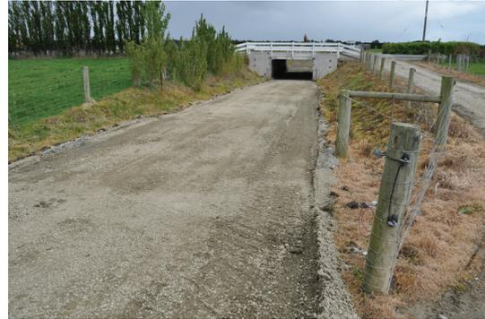
Remove overburden, apply GAP20 base aggregate and roll
